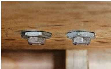
Figure 36: Fastened silencers
