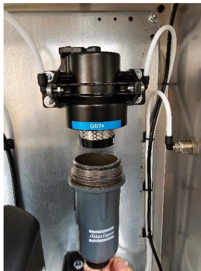
Figure 28: Filter bowl removed showing old QD7+ filter
