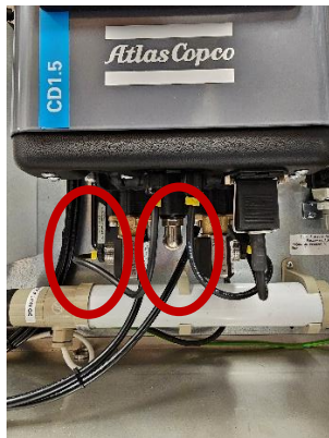
Figure 50: Solenoid valves location
