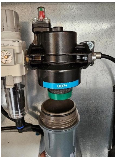
Figure 21: Filter bowl removed showing old UD7+ filter
