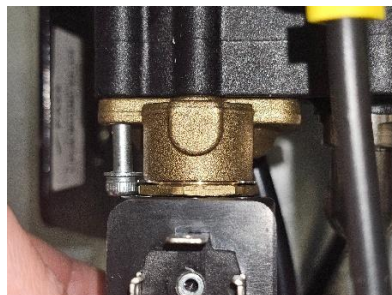
Figure 57: Solenoid seated without gap or diaphragm pinching
