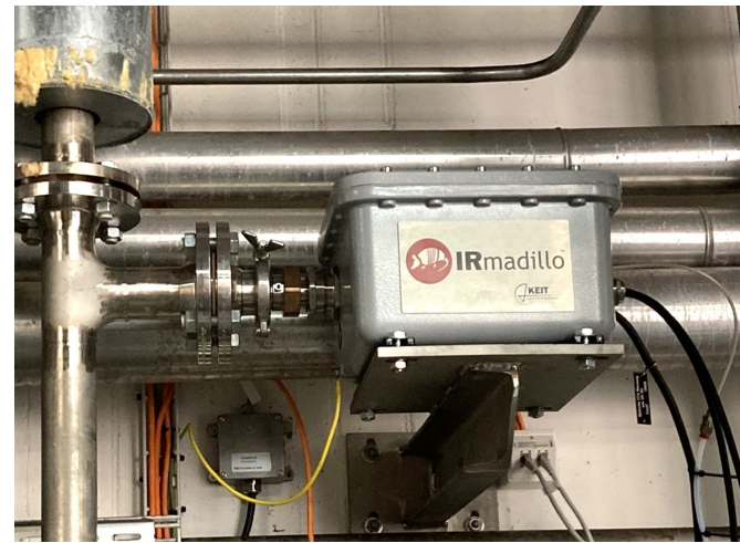
Above: The IRmadillo installed on the inlet of the centrifuge at Florin AG
