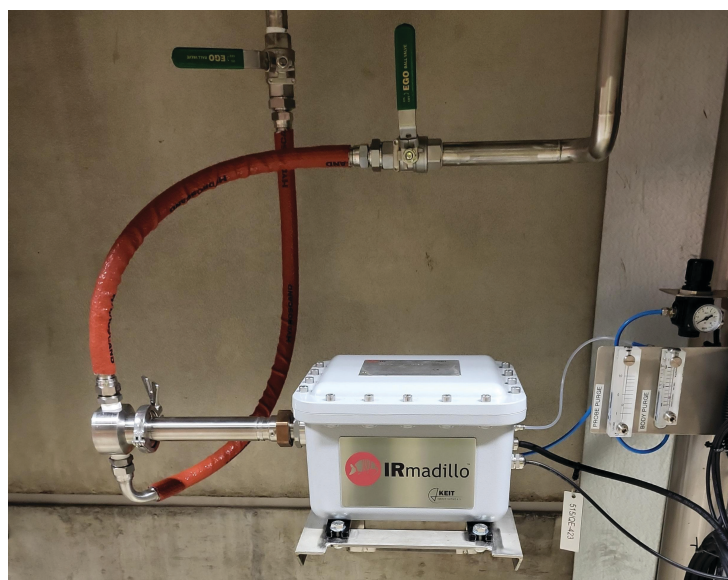
Photo: Installation of an IRmadillo instrument into the outlet stream from the mill's weak black liquor tank, using a flow cell for continuous process measurement.
