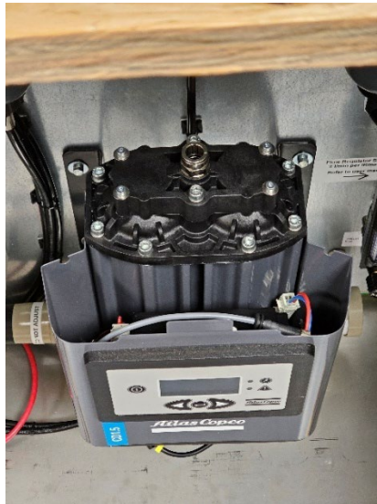
Figure 40: Cover removed exposing desiccant chamber cap
