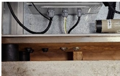
Figure 33: Exhaust silencers location
