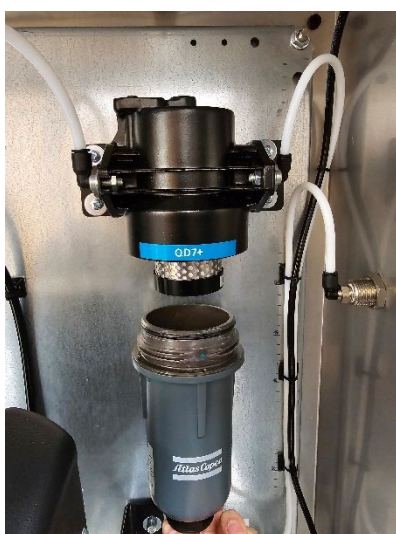
Figure 28: Filter bowl removed showing old QD7+ filter
