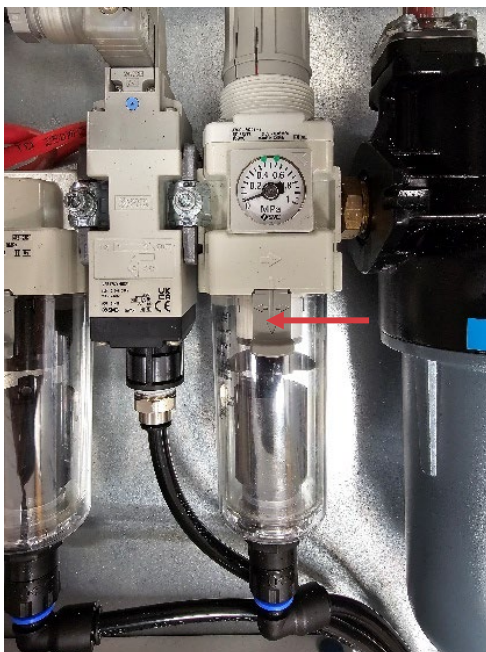
Figure 18: Maintenance complete, unit reassembled
