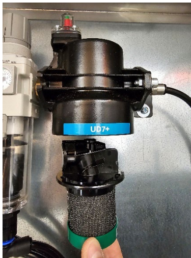
Figure 24: Inserting new UD7+ filter
