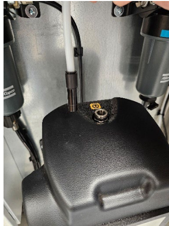
Figure 38: Removing push fit piping
