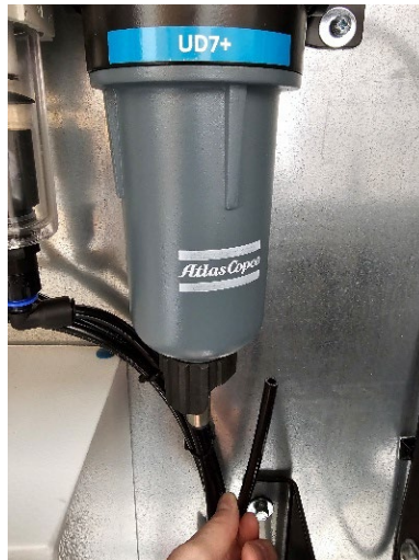
Figure 20: Push fit drain removed
