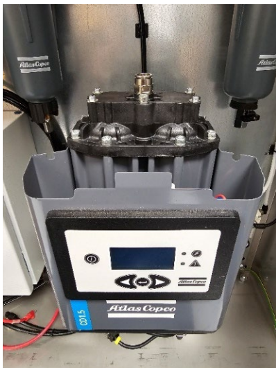
Figure 48: Cap fastened with screws
