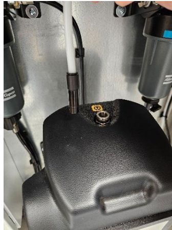
Figure 38: Removing push fit piping
