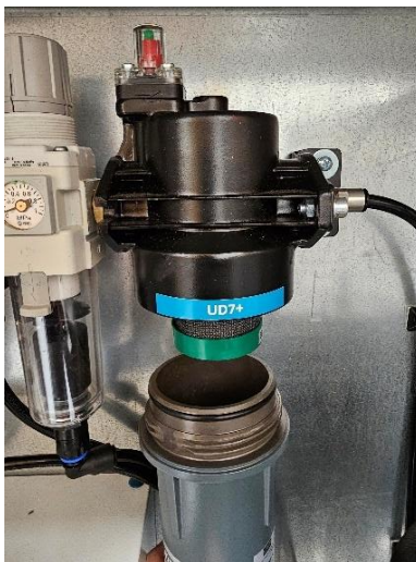
Figure 21: Filter bowl removed showing old UD7+ filter
