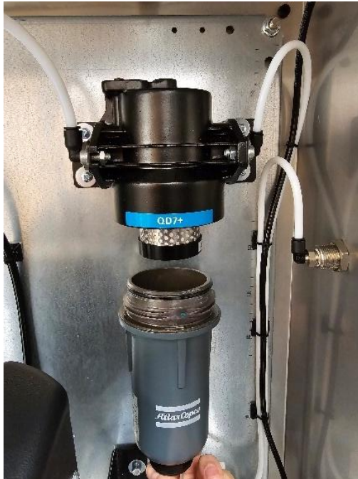
Figure 31: New QD7+ filter inserted
