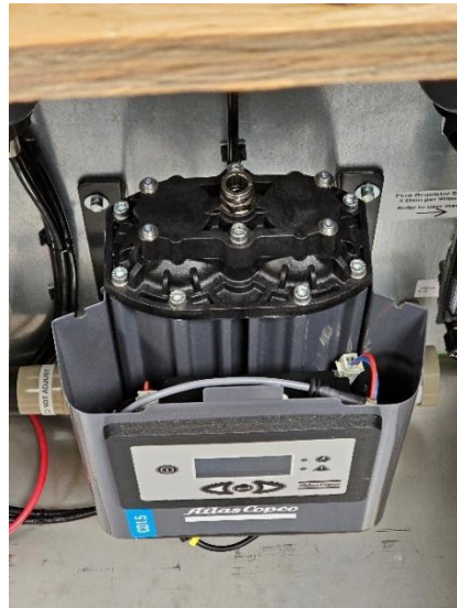
Figure 40: Cover removed exposing desiccant chamber cap
