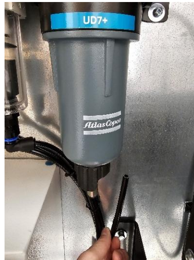
Figure 20: Push fit drain removed
