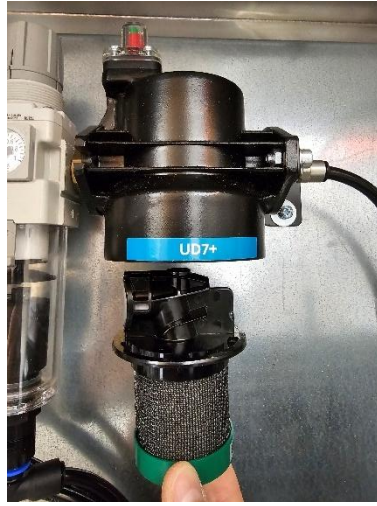
Figure 24: Inserting new UD7+ filter
