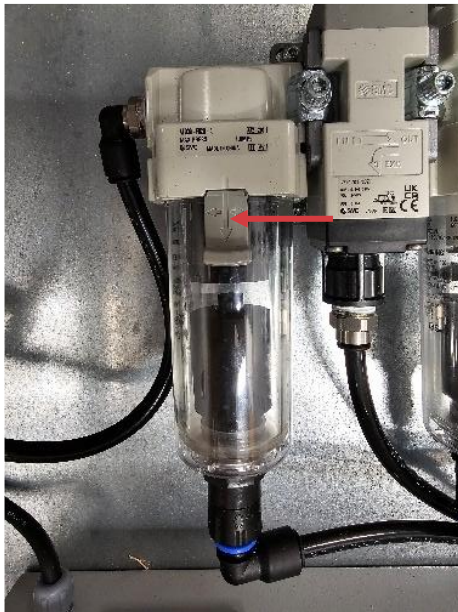
Figure 12: Maintenance complete, unit reassembled
