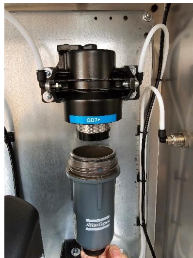
Figure 28: Filter bowl removed showing old QD7+ filter
