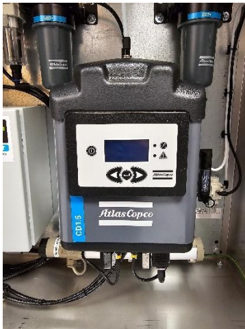
Figure 37: CD1.5 desiccant dryer
