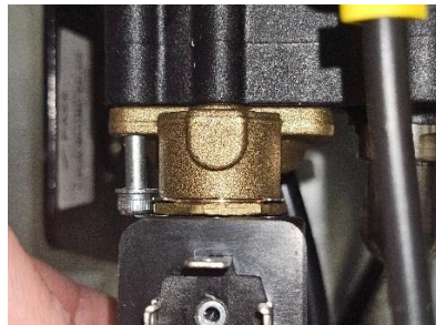
Figure 57: Solenoid seated without gap or diaphragm pinching
