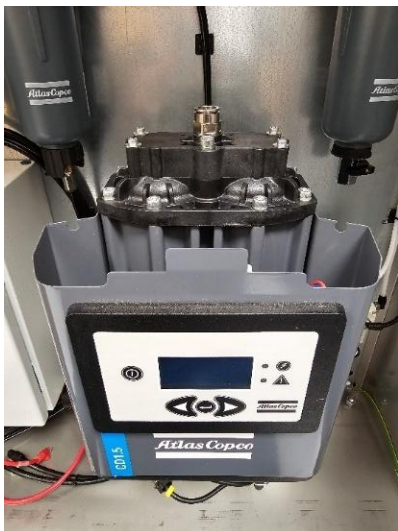
Figure 48: Cap fastened with screws
