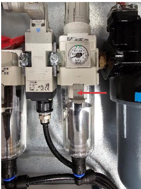
Figure 18: Maintenance complete, unit reassembled
