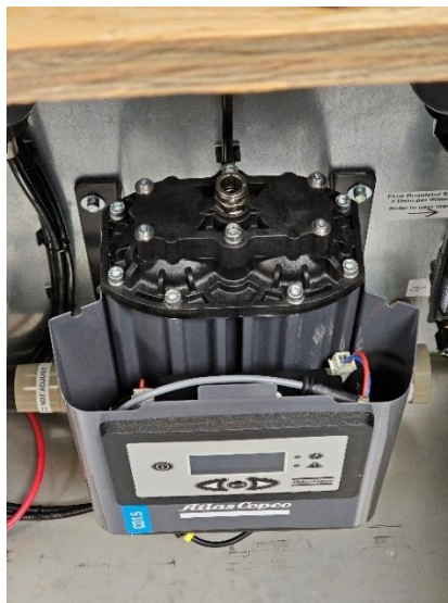
Figure 40: Cover removed exposing desiccant chamber cap
