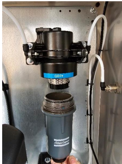
Figure 28: Filter bowl removed showing old QD7+ filter
