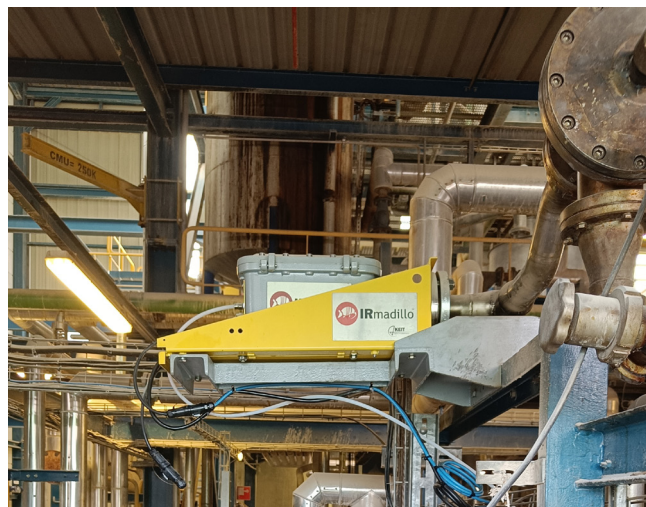
Figure 1: IRmadillo installed after the centrifuge to monitor the degumming process.
